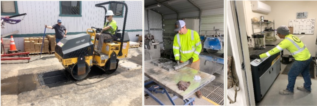
Figure Source: Granite Construction
