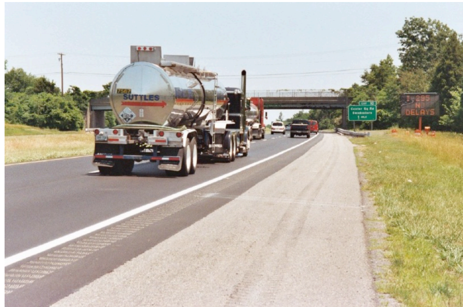
1" Thick Lift with or without milling
