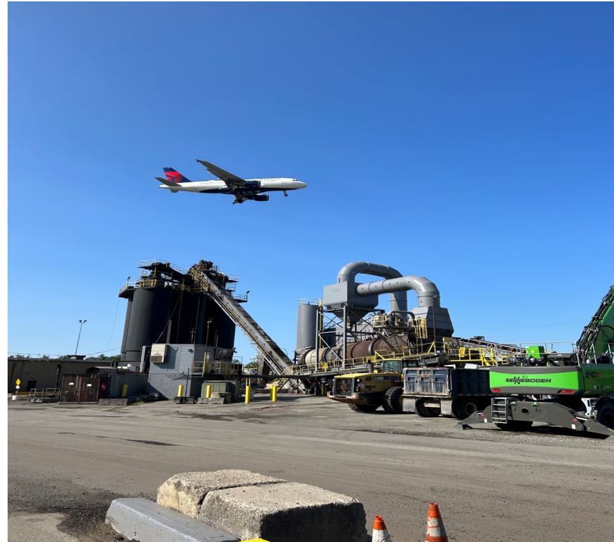
Flushing Asphalt, Flushing, NY
