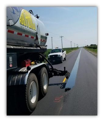
Placed by pressure distributor with mechanical agitation in tank
