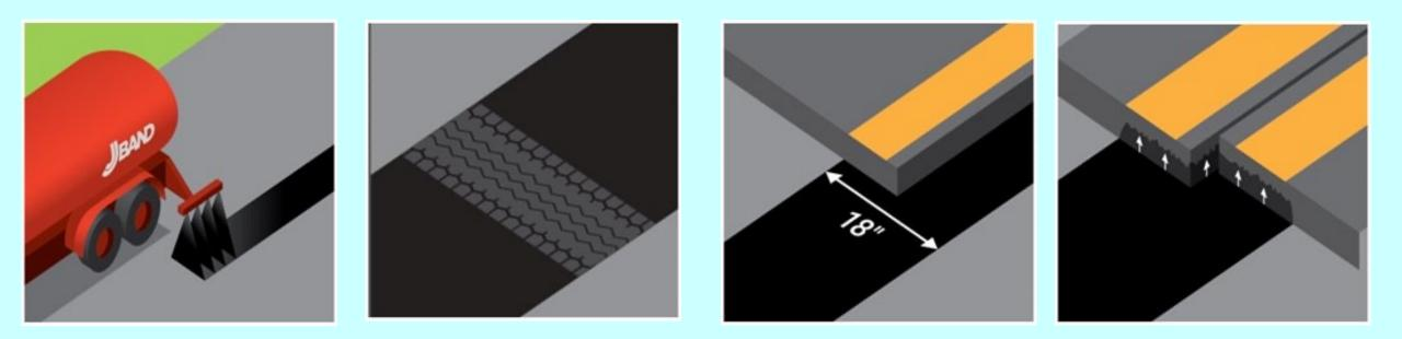
Apply a heavy band of polymer modified binder in the area where the new paving joint will be placed. Fast acting, the road is ready for construction traffic, keeping the installation process efficient and traffic flowing. Place the first paving pass over half the width of the band of polymer modified binder Polymer modified binder migrates into the HMA at the joint
