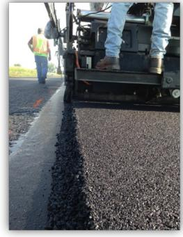
1<sup>st</sup> pass covering half VRAM width. Joint density testing not required within 1 ft from joint.
