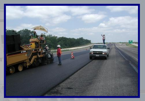
Initial research included the use of a thermal camera operated by a researcher in the back of a pickup truck. In addition to obvious safety considerations, this initial method was found not to be practical. A series of infrared images had to be manually combined to produce a complete profile. Distance and position data were also difficult to incorporate.
