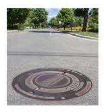
SELFLEVEL assembly floats with the roadway, keeping the surface smooth during settling and frost heave.
